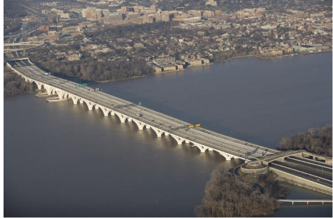
Woodrow Wilson Bridge, looking northwest over the Potomac River toward Alexandria, Virginia. Traffic flows freely in this photo, but several months earlier, the final stages of construction on the new bridge severely constricted traffic in both directions. Photo: Virginia Department of Transportation, December 14, 2008, via Flickr .
